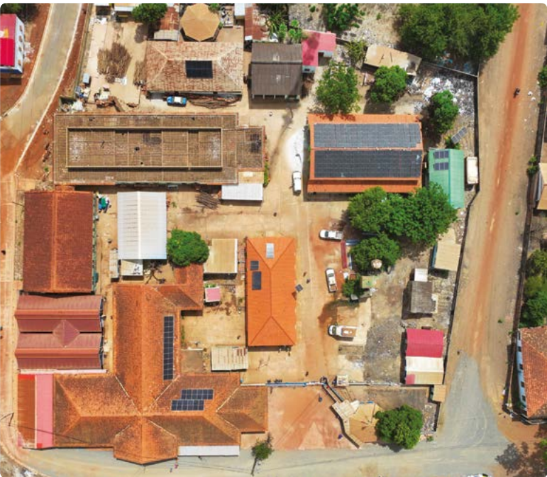
Aerial photograph of the refurbishment works at Bafatá Regional Hospital
