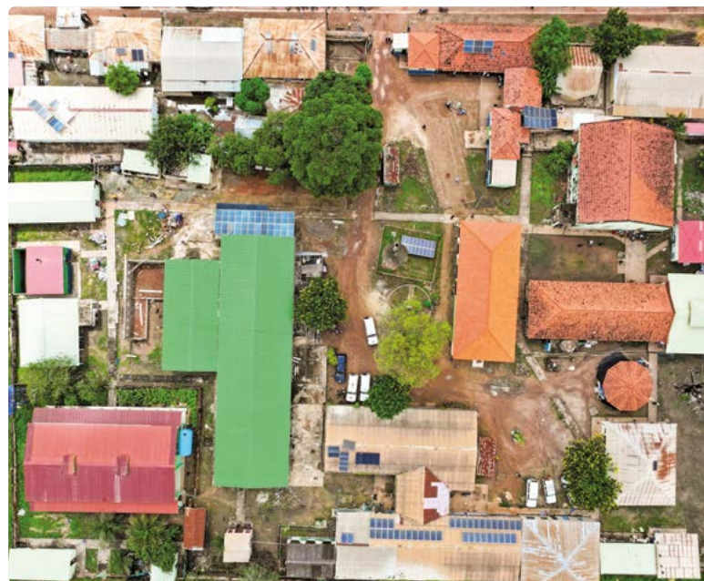
Aerial photograph of the refurbishment and construction work at Gabu Regional Hospital
